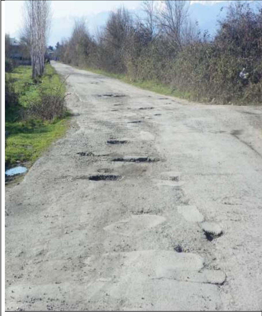
Attachment 2: Photos of the road to be rehabilitated
