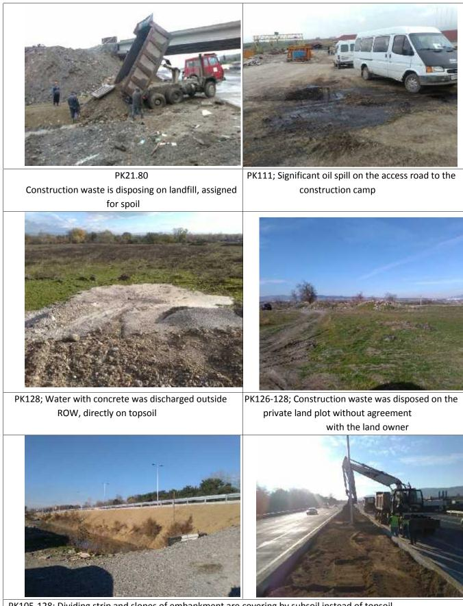
PK105-128; Dividing strip and slopes of embankment are covering by subsoil instead of topsoil
