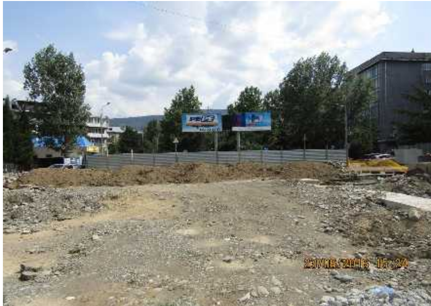
Photograph 1: Working area in good state
