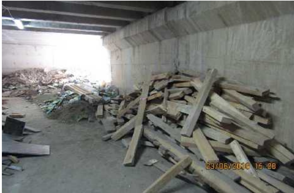
Photograph 3. Waste disposal inside the tunnel
