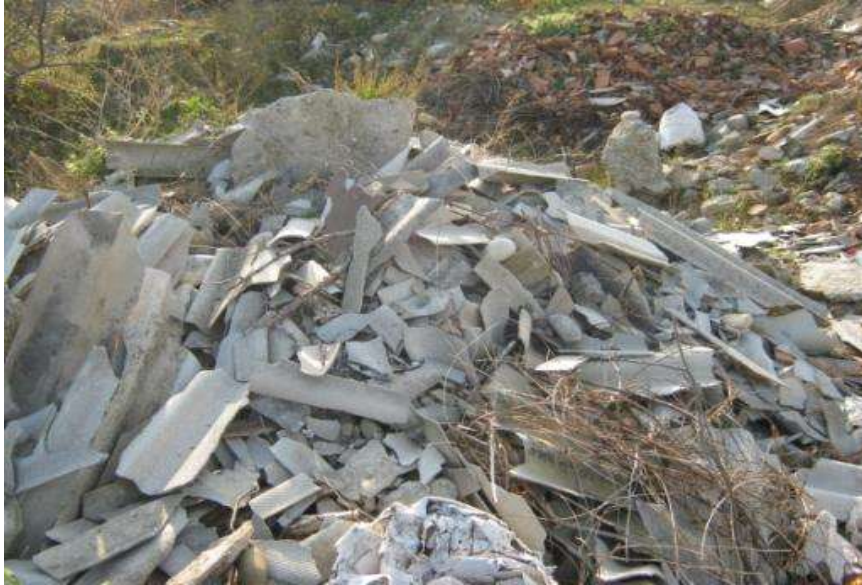
Site 3 – Debris of asbestos cement tiles dumped along the internal road.
