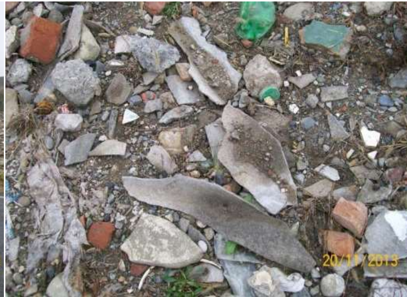
Site 5 – Typical waste dumped in the limits of the site. Asbestos cement roofing tiles dominate.
