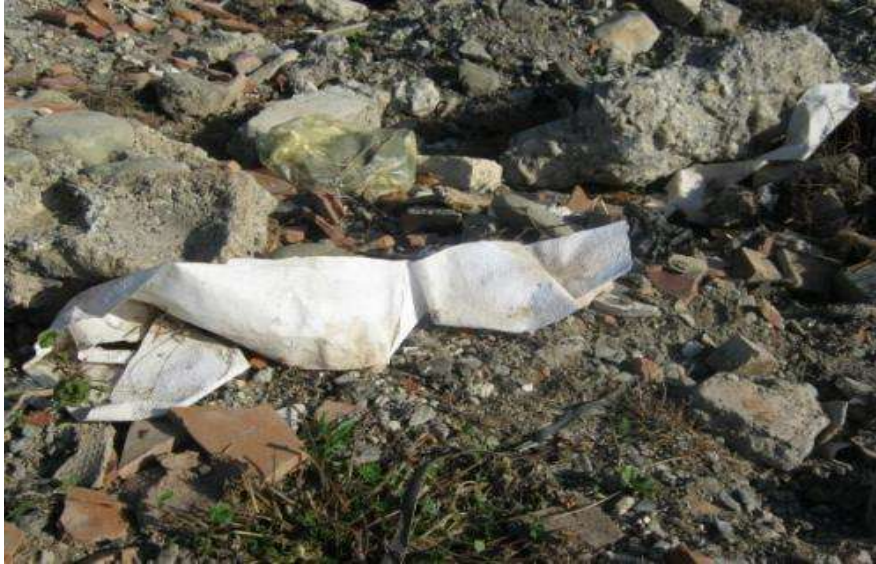
Site 1 2 – Typical waste: ceramic tiles, asbestosconcrete and tile fragments. White insulation material on the foreground.
