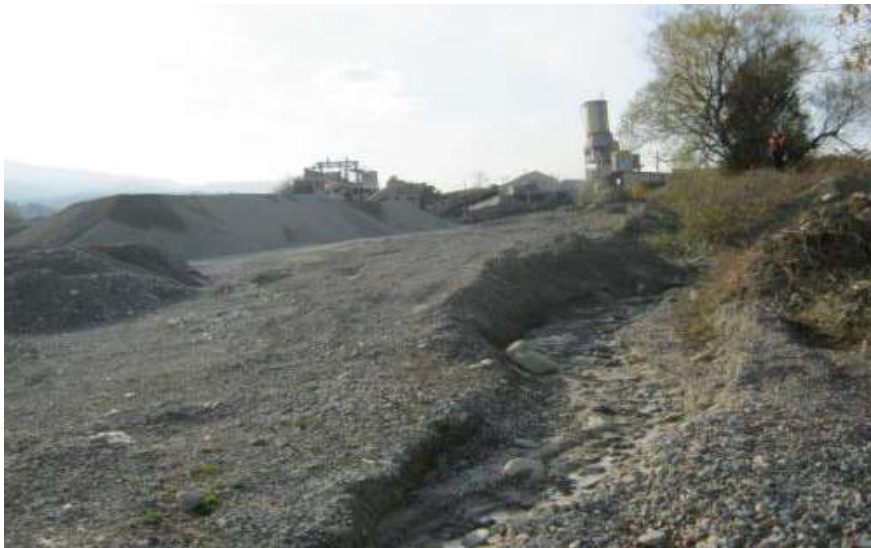
Inert material production facility west to the project site. Gully formed by waste water flow from production site.
