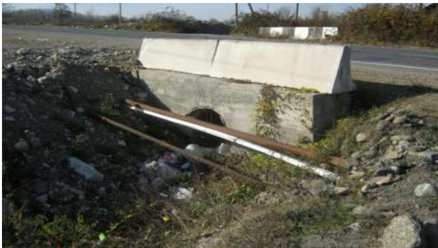
Site 1– Drainabe pipecap in the mid section of the area; 50 and 100mm water pipes and electric cable (with white insulation)in the middle area.
