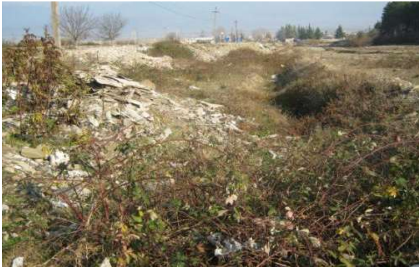
1.5 m wide, 0,8m deep trench along the site.
