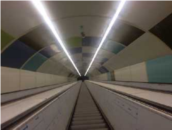
Escalator is installed
