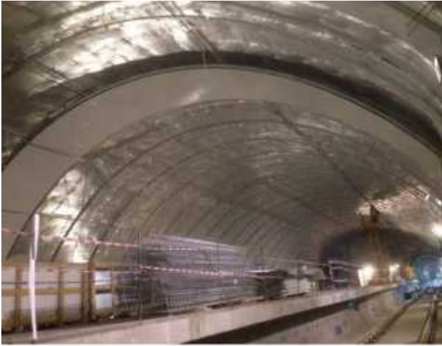
Installation of superstructure steel panel in platform
