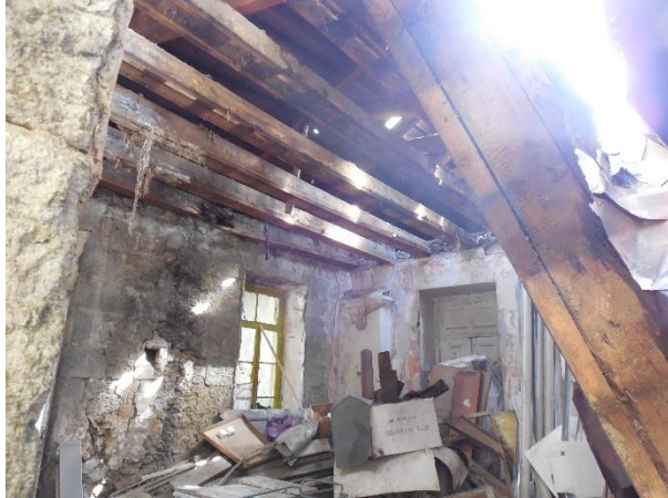
Figure 5. Apartment on the rear façade
