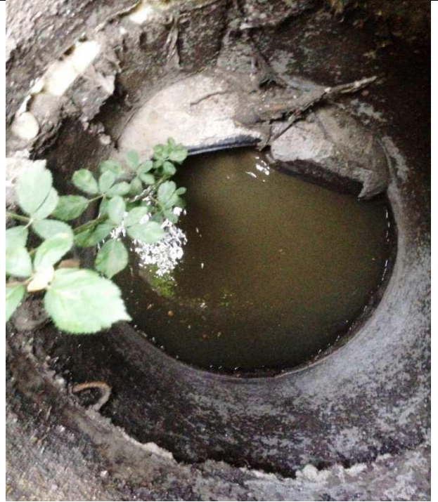
End of main trunk leading to Irrigation Channel (Akhmeta to Dedoplistkaro) at Alazani Boulevard (the sewer ends after further 50m in a flooded pit hole)
