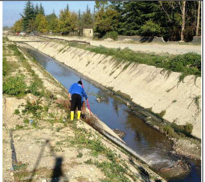
Telavi main sewer draining to irrigation channel
