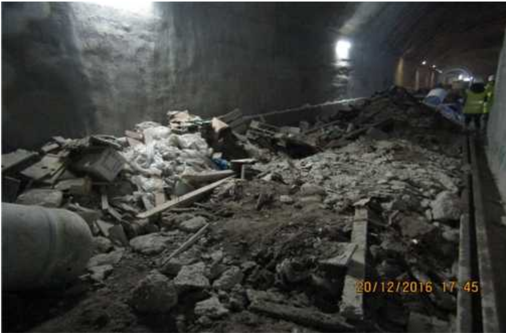
Photo 1: Specific waste disposal inside the tunnels. Plastic wood and debris are being conveniently separated in this point
