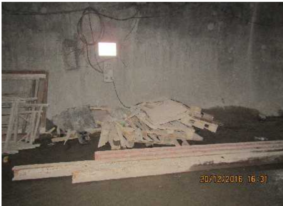
Photo 2: Waste disposal inside the tunnels. Adequate Wood separation and compilation
