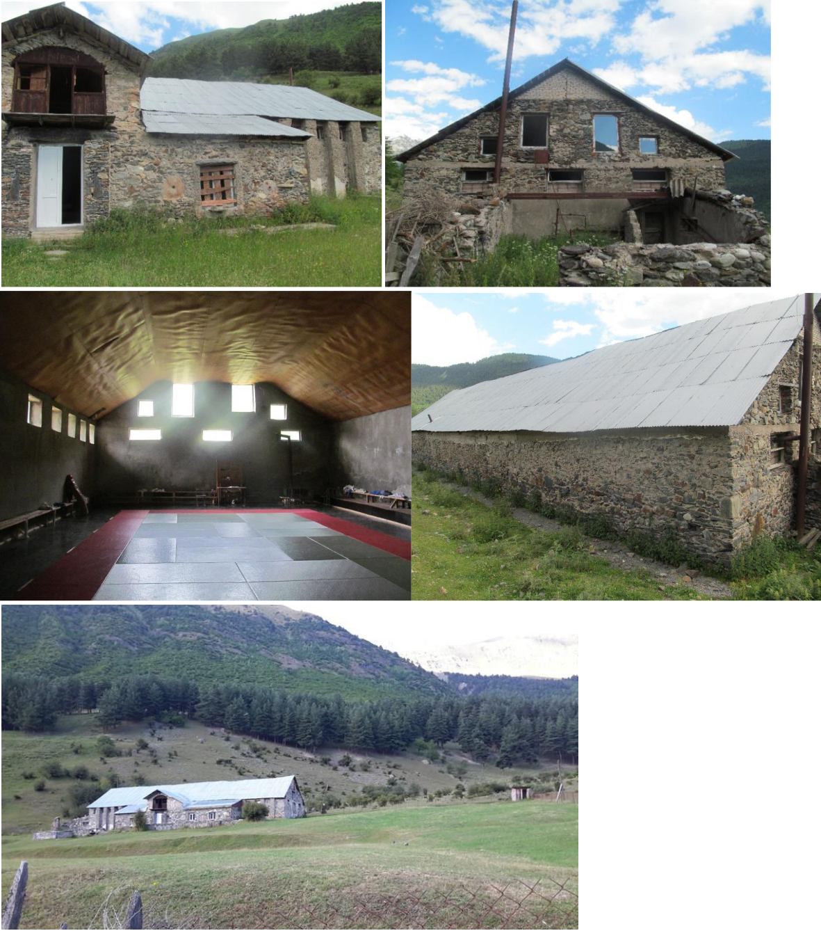
Figure 3. Pictures of the existing building
