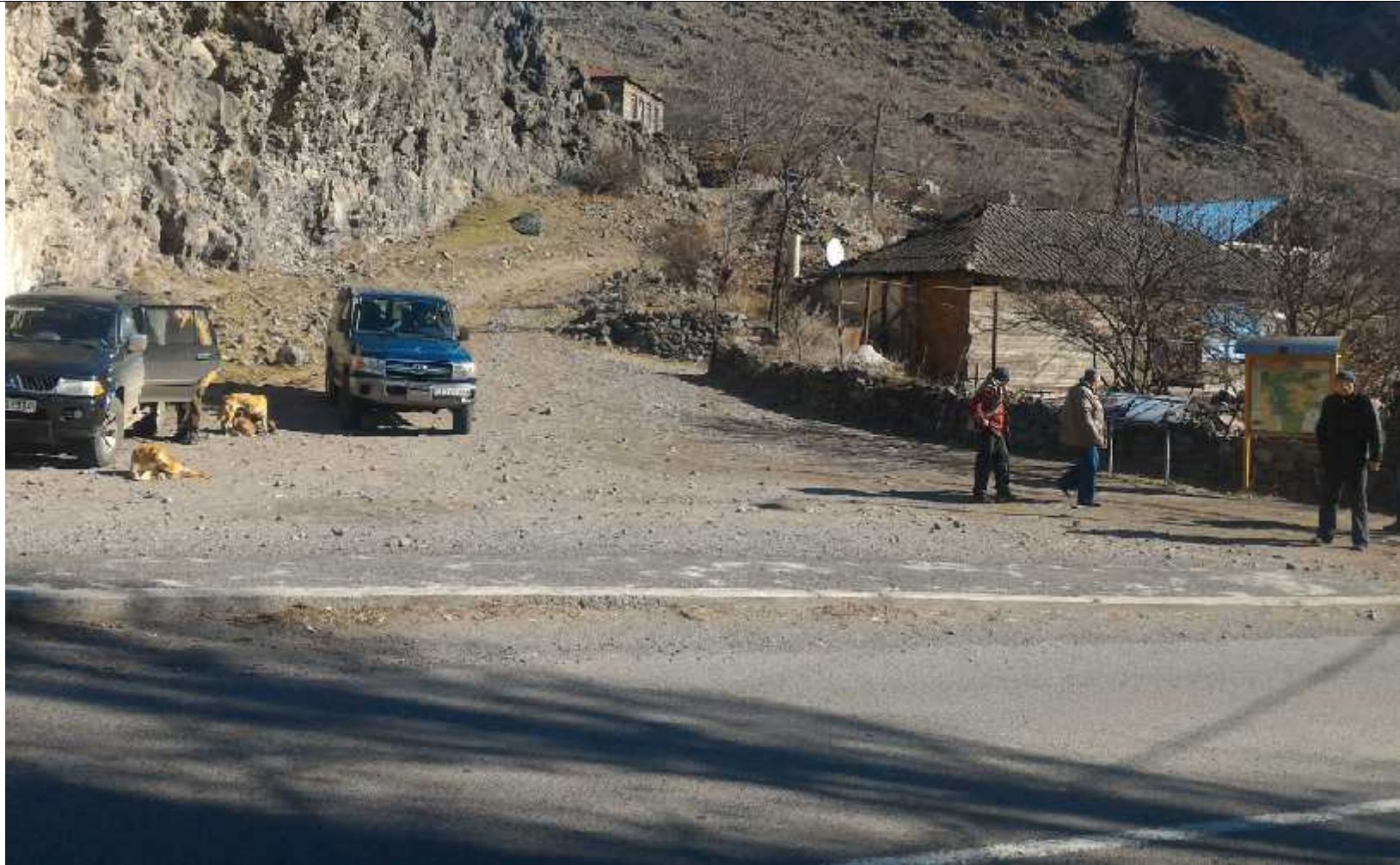
The road and fences to be rehabilitated
