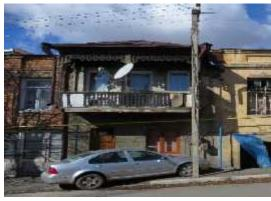
House # 20 (Cultural Heritage Monument<sup>5</sup>) - Twostorey brick building with wooden balconies. The entire façade will be cleaned from poor quality and damdamaged plaster, the doors and windows will be replaced, the open balcony will be restored (the most part of the balcony will be replaced with new ones), the facade will be plartered with sand-cement mortar. Roof plankins and gray tin cover of all three houses will be replaced. There will be arranged a basalt socle on the façade.
