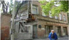
elements of balcony and staircase. The doors and windows will be completely changed, stained glass windows and basement on the first floor will be cleaned, and parapet will be restored.
