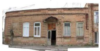
low parapet on the both sides of the street, it is covered with usual black tin. The SP envisages removal of the existing roof and arrangement of the dark tin sheets on the the new wooden structure; Cleaning of the façade using sand-jet blower, replacing of the existing doors and windows with new wooden doors and windows, restoration of the entrance
