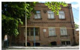
a large basement in the building which has entrance from Rustaveli Street. The project includes removing of the existing roof cover and arranging a dark tin layer on a new wooden construction of the ceiling rafter. Restoration of demolished parts of the building such as: brick arche and doors at
