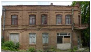
painting, restoration of the wooden decorative elements from the yard, and replacing of the missing part with the new one, dismantling of the ugly staircase going to the second and arrangement of new wooden one using the existing wooden decorative elements. The wooden planks and tin cover will be replaced with new one.
