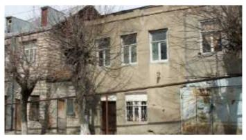
dismantling the existing doors, windows and metal gate; removing the rebuilt parts of doors' and windows' openings on the first floor; removing the old tin cover of the roof and the water drain pipes; dismantling the damaged wooden structures and plancking of the roof; Cleaning the façade from old plaster using sand-jet machine. Reconstruction works include: restoration of damaged wooden
