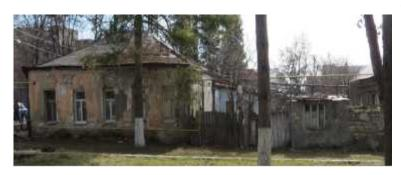
The SP envisages the rehabilitation of the building façade and the replacement of the roof, namely: cleaning the facade from the remained plastering, restoration of plastered cornices, replacing doors and windows and canopies, dismantling of fence of the yard and the metal gate and
