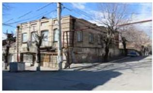
The two-storey building is built of stone and brick mixed masonry, and which later have been plasterd. The second floor is built with brick. The rehabilitation works include removal of the existing roof and arrangement of the dark tin layer on the new wooden structure of ceiling rafter. Removal of cement plastering on the first floor and restoration of the old masony, cleaning and restoration of the brick façade on the entire the perimeter of
