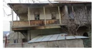
structures, rehabilitation of the balcony and glass galerry – rearrangement of wooden columns and railings, fabrication and installation of new wooden rail post and and windows glass gallery. Complete replacement of ceiling planking and floors of the balcony. The replacement of doors and windows is not provided by the project. They will be cleaned, processed and painted wih oil
