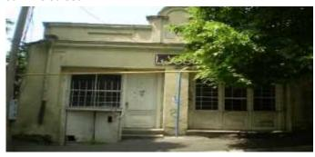
At present, the house # 16 (Cultural Heritage Monument<sup>4</sup>), is a one-storey with a basement, and requires repair and restoration of the façade of and plastered cornices, replacement doors and windows, and restoration of staircase passing to the facase and leading down to the basement (basalt slabs).
