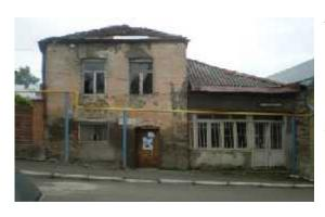
The SP includes rehabilitation of building façade and replacement of the roof. As of today, one part of a House # 13 is a two-story ant the other part – one-storey. The SP provides works for removal of bad-quality plaster and re-plastering of entire façade of the bulding with sand-cement mortar. Replacement of doors and windows and restoration of stair steps. The roof planking and tin cover will be replaced with gray color tin sheets.
