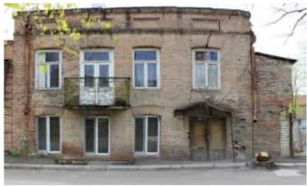
House is a two-story building, constructed with Old Russian brick and covered with ordinary black tin. The project envisages replacement of existing roof and arrangement of dark tin roofing. Replacement of wooden doors and windows, restoration of the wooden entrance door in its original form. The later rebuilt part will rearranged with new metal structure, which will strengthen the cracked wall, the exterior
