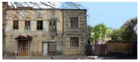
the façade from existing plasteering, replacement of doors and windows, re-built a wooden balcony (similar to balcony of of the house on Erekle II Street # 9) from Erekle II street side. There is also envisaged
