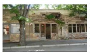
The house is a one-storey brick building, with backyard. In the left corner of the bulding from the Shamanauri street is located a store, after it is a living area, and in the rest area of the bulding floors and ceiling is demolished. Building was reconstructed several times and plastered.
