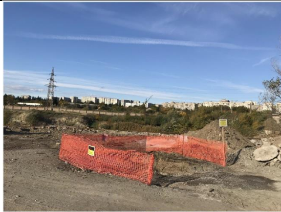
Photograph No. 9 Concrete washing pit
