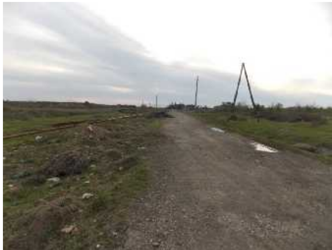
Picture 4.2.3. Pressurized Sewer Corridor
