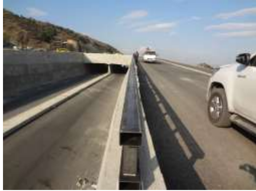
Tunnel Guard Rail Installation at PK 98+24.
