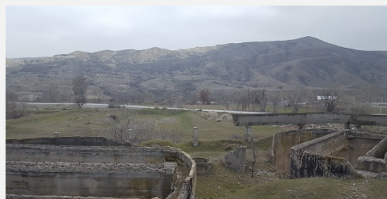
Photo 1: Remains of the old sewage treatment plant
