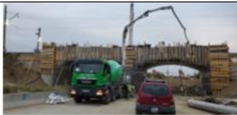
Railway underpass construction works: Concrete pouring
