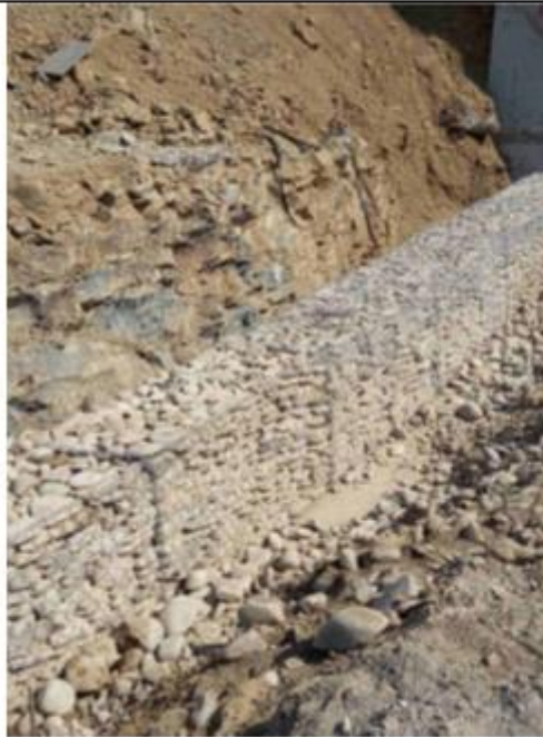
Gabion construction works on the Railway underpass
