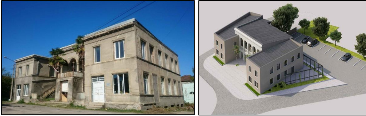
Figure 2: Existing situation and render, building of village Velisthikhe local administration office
