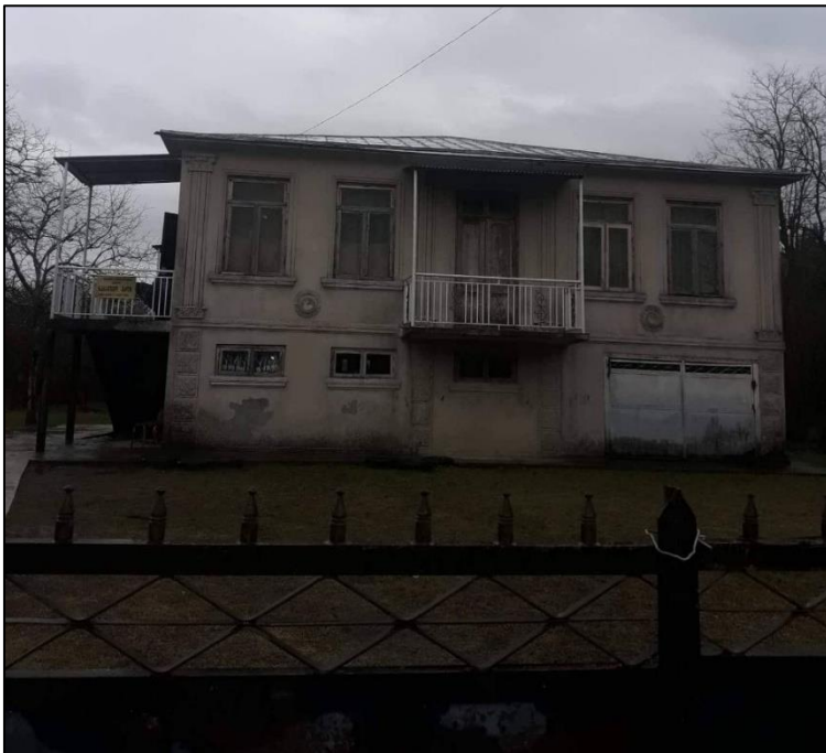
Figure 5. Building of the existing kindergarten
