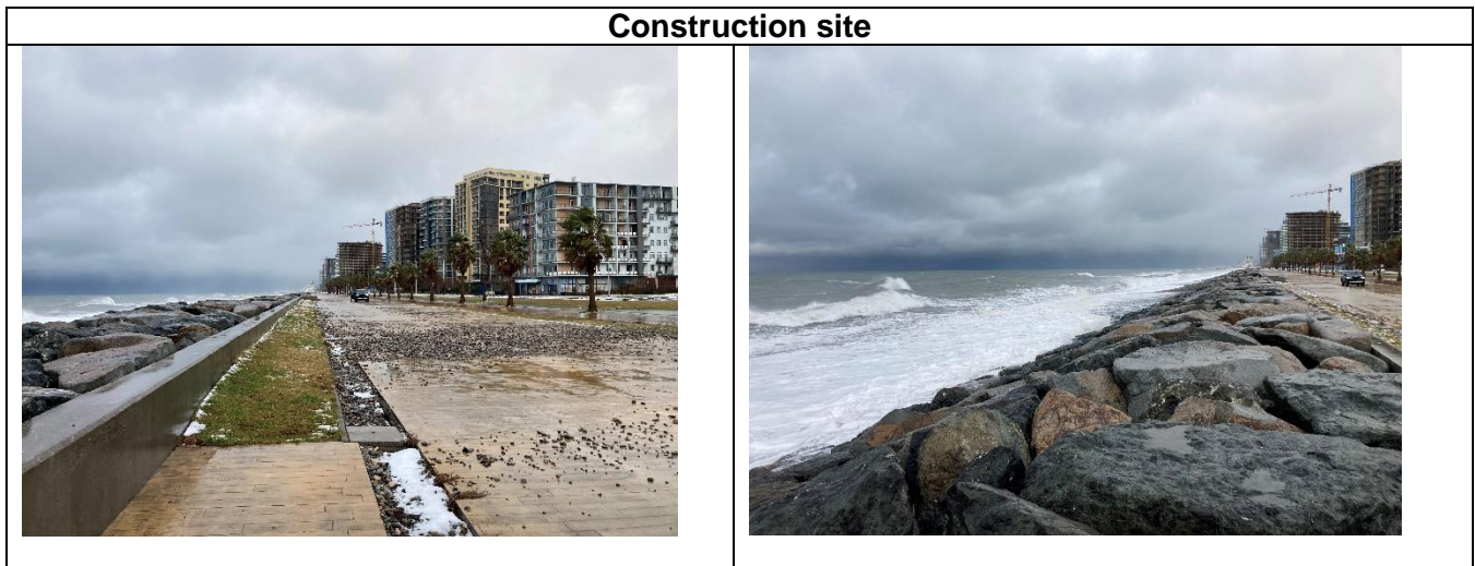
Figures 1-2: Photo Materials of the construction site
