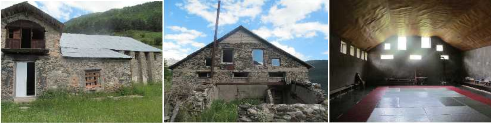
Figure 2. Pictures of the existing building
