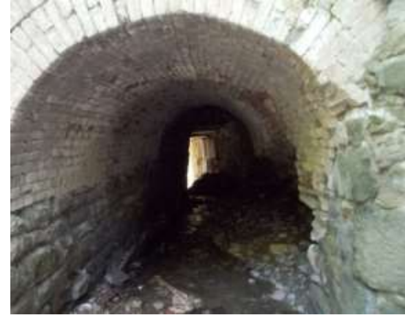
Ruined wall, view from entrance
